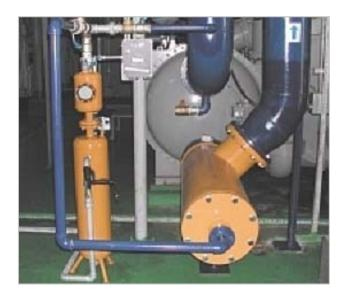
ATCS-Industrial Automatic Tube Cleaning System for Industrial Plants and Power Stations
